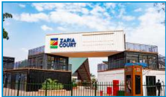
REAL CONTRACTOR, RWANDA, SHOPPING MALL
